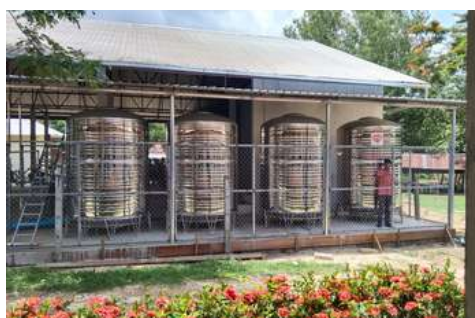
RFD room after completion
